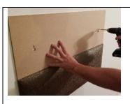
Place the template on top of the installed panel and mark the position
