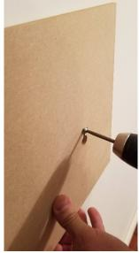
Tighten the screws so that the template is pressed against the wall but has enough space to move up and down
