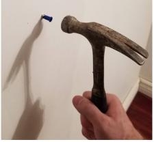
Hammer the anchor into the wall to make it flush
