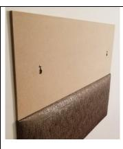
Once the second position has been marked, drill 1/4 of inch for anchor placement, insert the anchors, drill in the screws and install the template. You may refer to step #8
