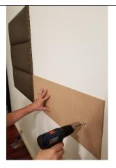
Press the template firmly next to the installed leather panel and mark the location (See step #2)
