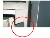
The glass panel is hooked by 2 hooks on each side.
